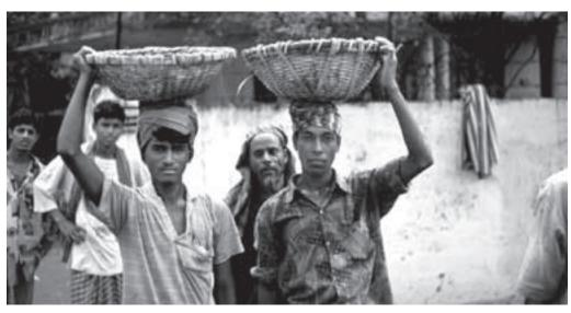
Labourers at a road work site in Dhaka carry materials for making concrete mix in the baskets on their heads. In the absence of electrical and mechanical equipment, manual labour is required. The work is physically exhausting: the strain on the head and neck takes its toll as the years pass.
