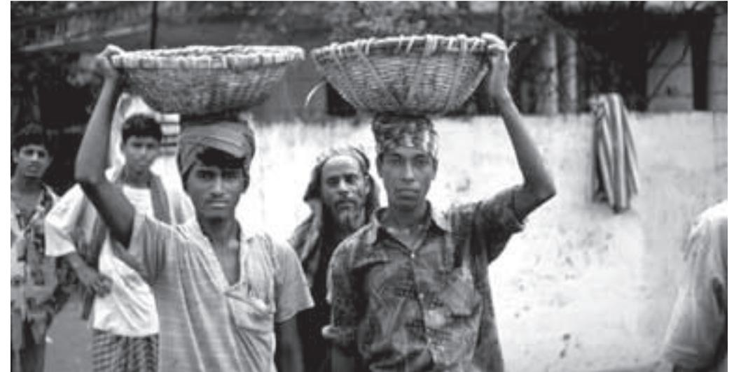
Labourers at a road work site in Dhaka carry materials for making concrete mix in the baskets on their heads. In the absence of electrical and mechanical equipment, manual labour is required. The work is physically exhausting: the strain on the head and neck takes its toll as the years pass.
